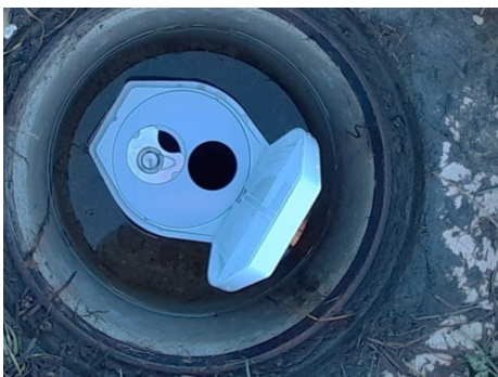
Well in manhole, use of intermediate ring
